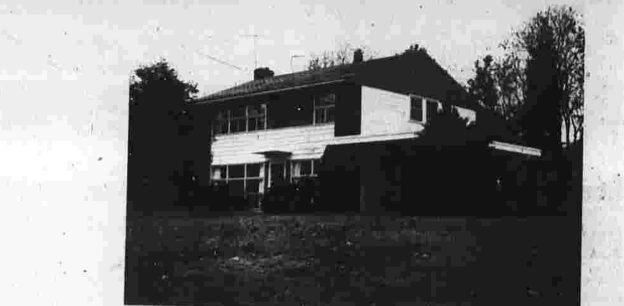
The McCandless home featuring extensive window area
