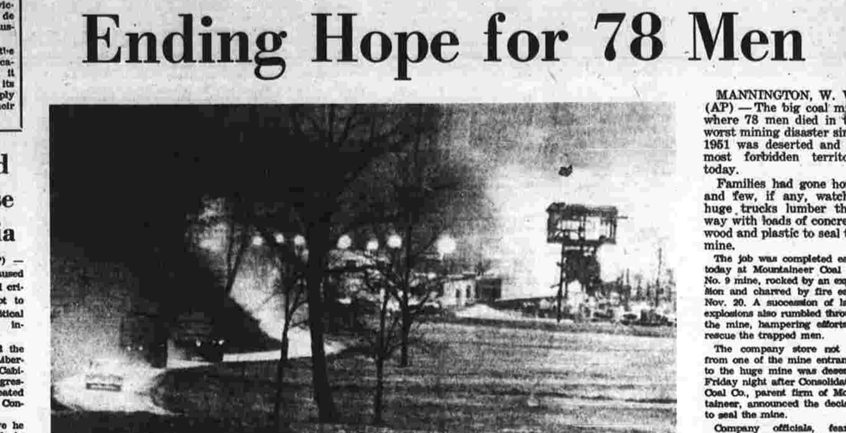
Huge dump trucks loaded with gravel (lower left) approach the Llewellyn Portal of the Consolidation Co.'s No. 9 mine at Farmington, W. Va., at dusk yesterday.
